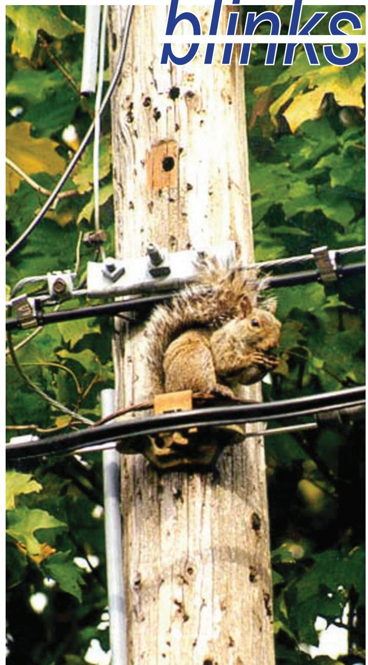
attributed to animals by installing insulated "bird wire" and wildlife protection devices to prevent animals and birds from making contact with electrical equipment. These devices are not only meant to protect the electrical system, but also the birds and animals.
