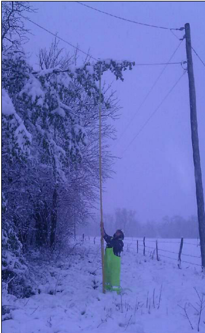
NO, YOUR EYES DO NOT DECIEVE YOU...Cooperative members woke up on the morning of May 3 to several inches of snow blanketing the area. Lineman Jesse Underwood works with a hotstick to remove a tree branch from a power line.
